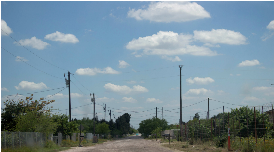
The lack of street and storm water infrastructure seen in a colonia north of Weslaco, Texas. Source: Danielle Zoe Rivera.
